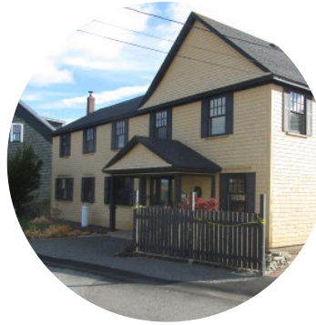
Zone 1 House: Incorporates traditional exterior components.
